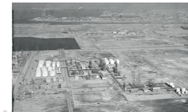
Nissan Petrochemicals Chiba Plant (1968)
