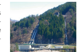
Miza Power Station
